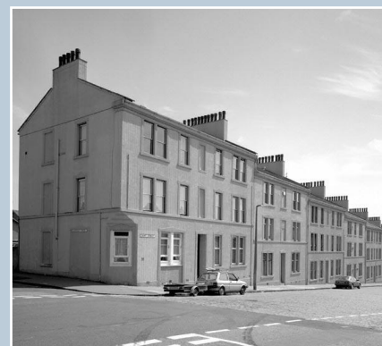
Mass concrete tenements in Dundee, cast insitu in 1874–5 by the Concrete Building Company for the Working Men's House Building Association. The buildings were renovated and a buff render applied in 1982–4. © Crown copyright: RCAHMS. Licensor www.rcahms.gov.uk .
