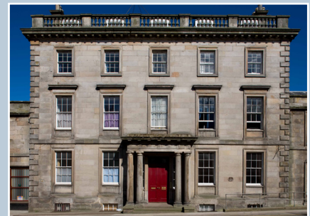
Central block of the former Fife Arms Hotel, Banff, 1843–5. The classical design places emphasis on the symmetry, proportions and detailing of the walls and reflects the functional hierarchy of the interior. Corniced windows indicate the principal rooms on the first floor; smaller windows relate to private or subsidiary rooms. The design maximises the architectural impact of the walls by hiding the shallow pitched roof behind a parapet. © N.Haynes.
